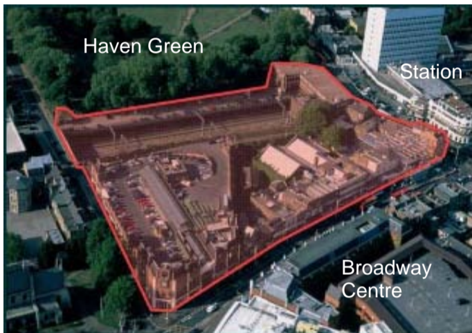
The Arcadia site from the air
