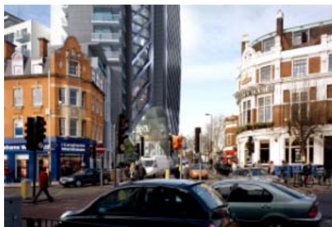
Base of tower from Ealing Broadway looking north
